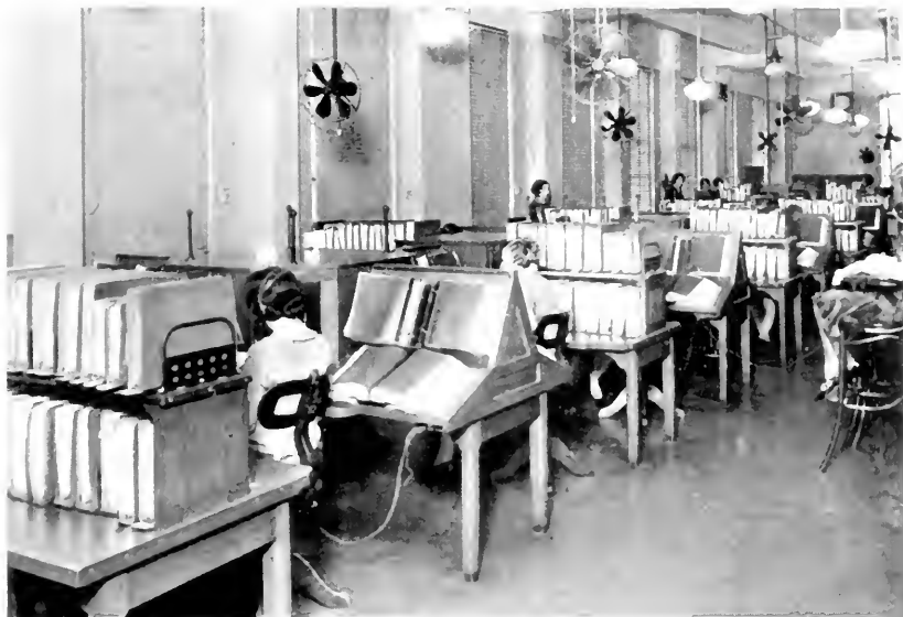
ONE OF THE TWENTY-FIVE INFORMATION BUREAUX IN THE AREA. CHANGES IN TELEPHONE NUMBERS ARE LISTED HERE PROMPTLY
